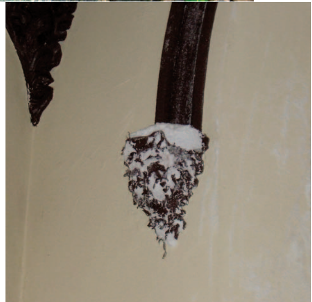
Top: This picture shows degradation of mortar on exterior of Renwick Chapel.
