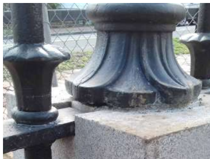
Restored post on a new base. Note the slot on the side of the base
