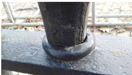
The bottom of a picket before epoxy
