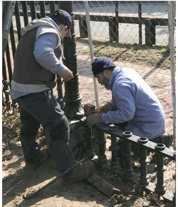
Fitting the bottom rail into an existing base
