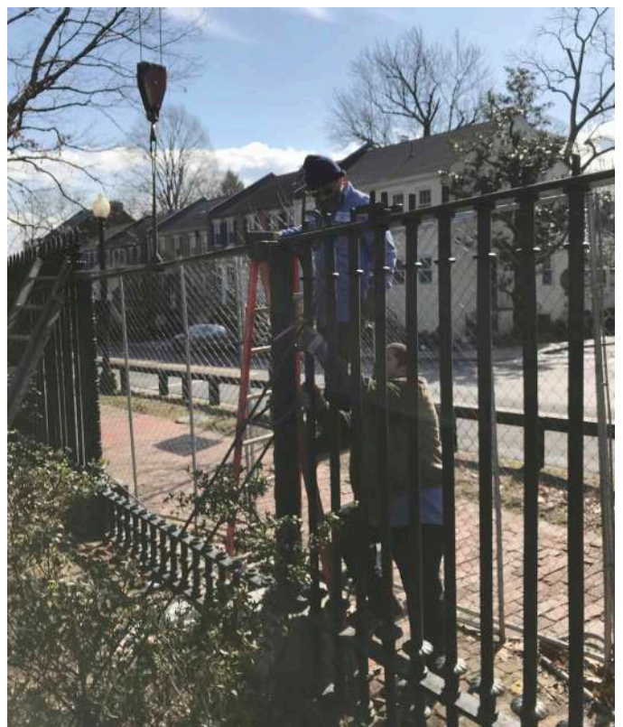
Setting pickets into the restored top and bottom rails
