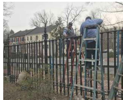
Preparing the pickets to accept the restored finials
