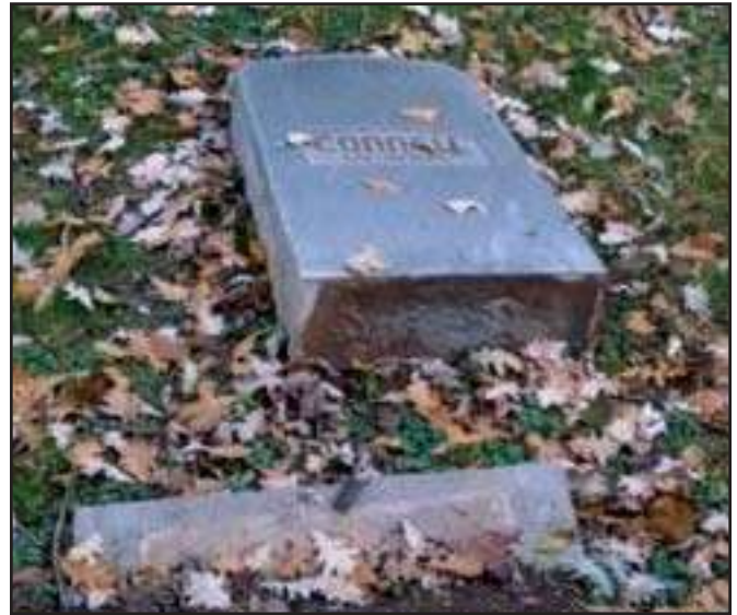
Above: Connell Monument Stone, Lot 508E, the monument stone fallen over; headstone completely detached from base.
