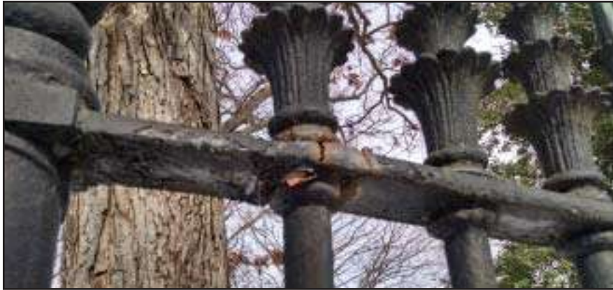
Picture C: Oxidation attaching the top rail and pinial
