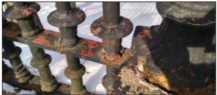
Picture D. Primer and rust showing near a deteriorated base
