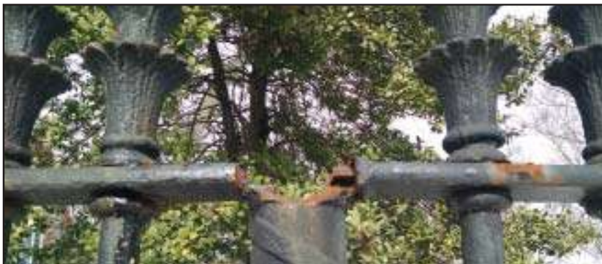
Picture E: The post finial connection completely failed
