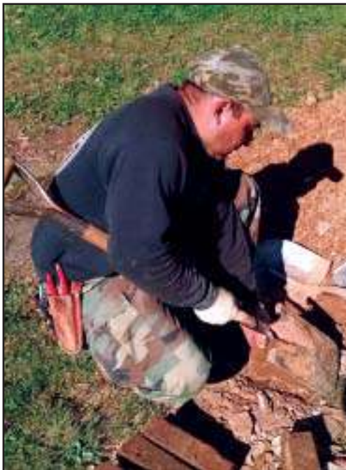
Staff member Jose Gurman working on the masonry catch basin.
