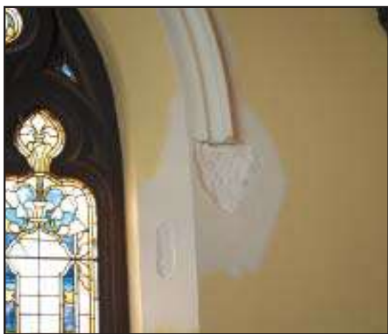
Plaster gothic ornaments that were damaged were replicated.
