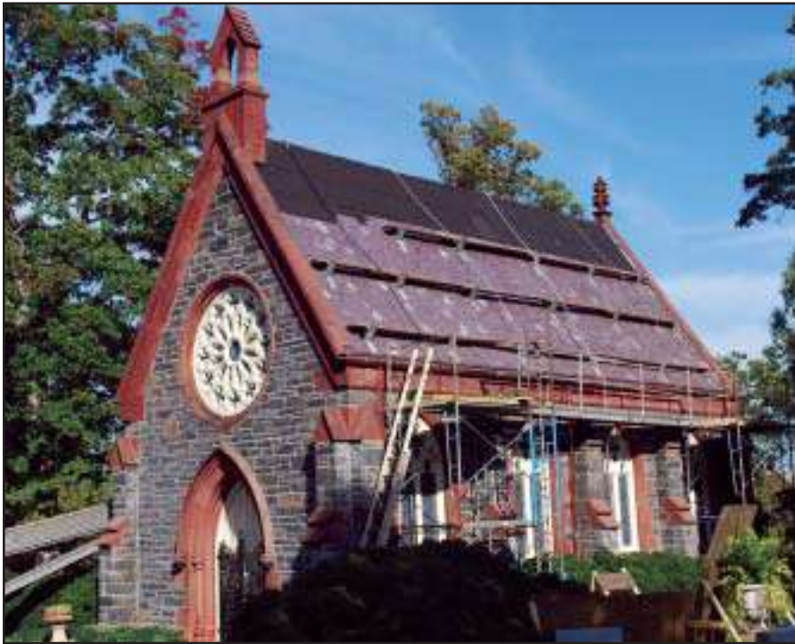
The entire slate roof was replaced after the old mortar was removed and replaced around the stone exterior walls. Photo by Dave Jackson.
