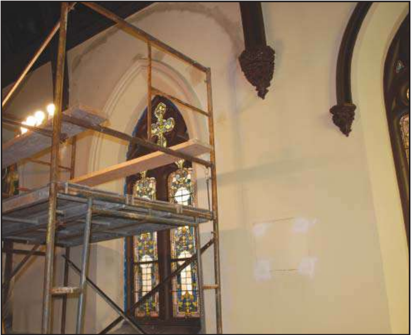
Work being performed by Washington Art Glass Studio. A number of small glass pieces had to be replaced in several windows. Supports were also added to the leading around the glass pieces to protect the overall strength of the windows.
