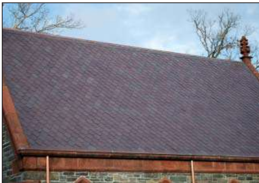
The new slate roof in, Wagner roofers carefully combed through the material to select only the slates which closely matched our requirement for purple, not variegated, and not a contrasting color.
