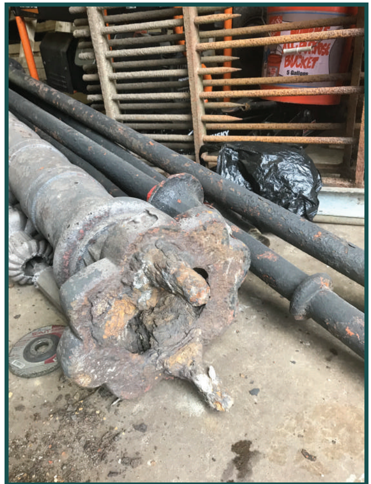
Bottom of a post that has been sandblasted. Welding repairs to come!
