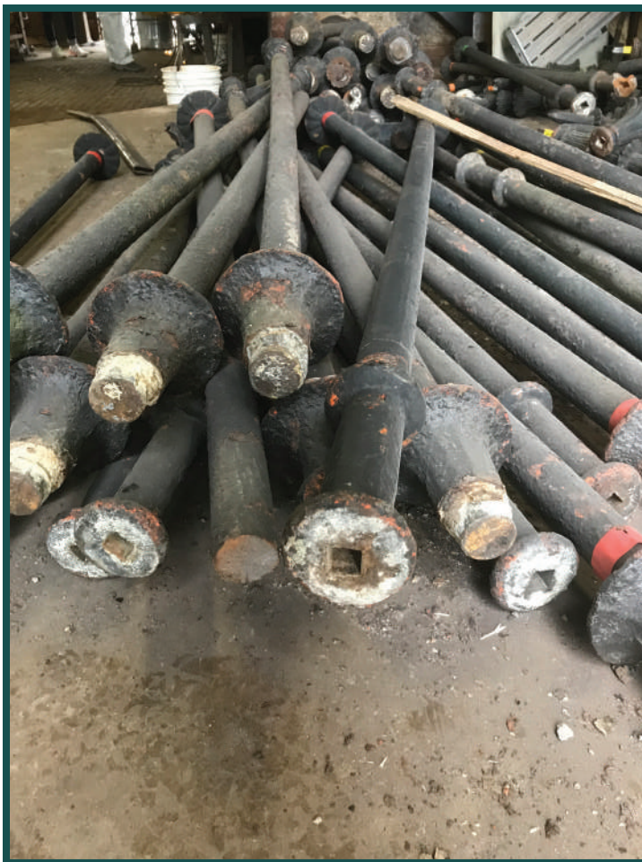
Bottom of pickets ready for sandblasting.
