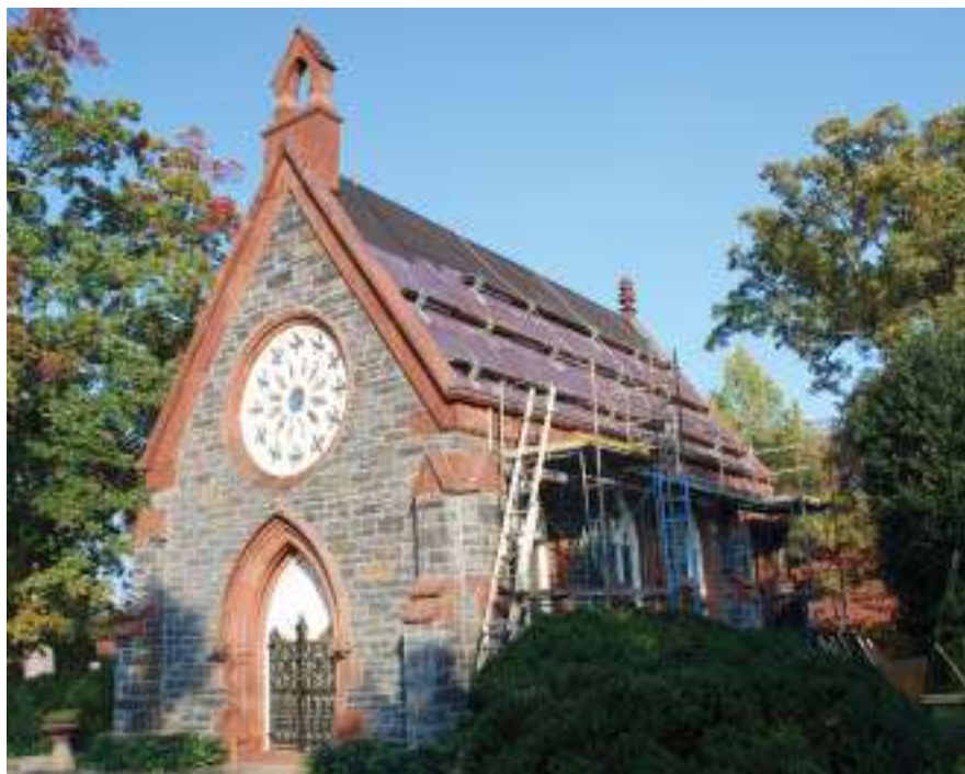
Slate roof replacement and other work underway on Renwick Chapel.
